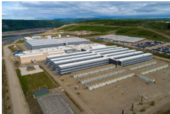
Site C Buildings
